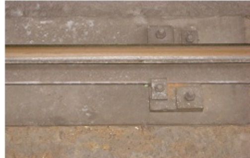
Landis Fastener - Plan View
