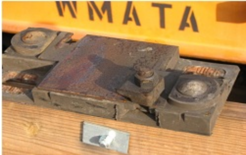
Hixon Fastener - Plan View
